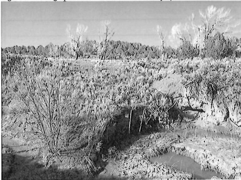
Figure 3 Leak. Notice sink hole next to creek. One option is to provide access at this location which would require grading back the banks to a 3:1 and place toe rock along the bank
