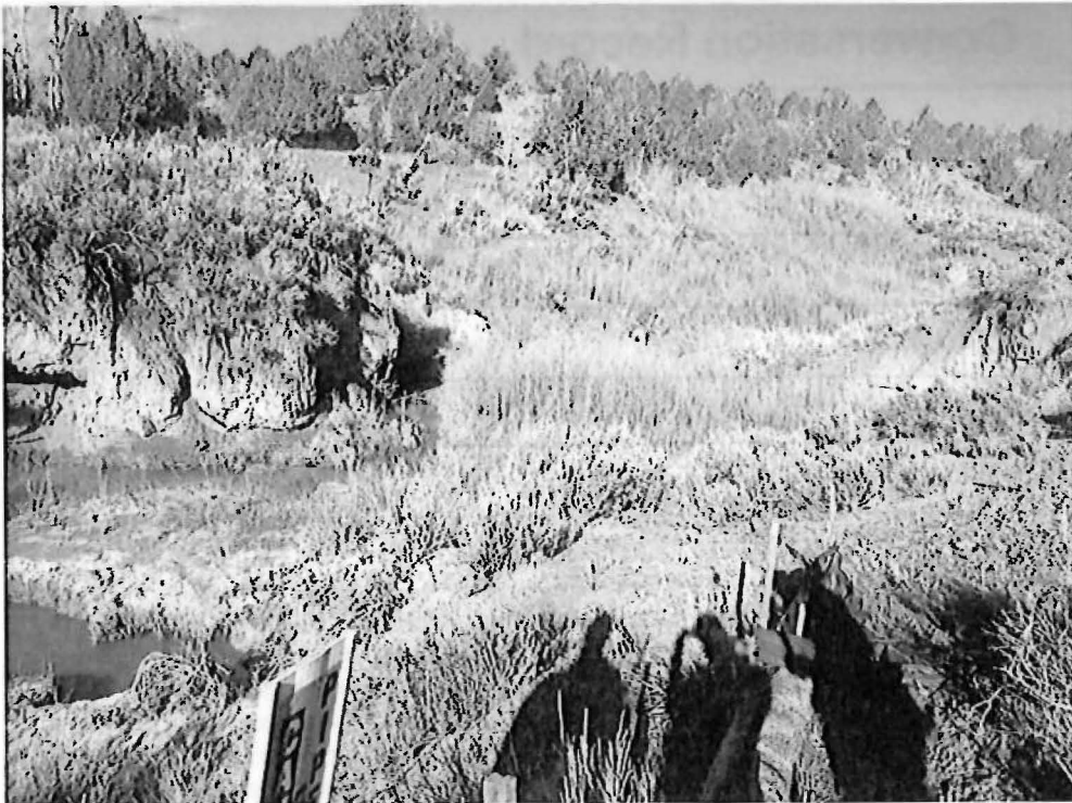
Figure 2 Looking upstream - stream immediately upstream of leak
